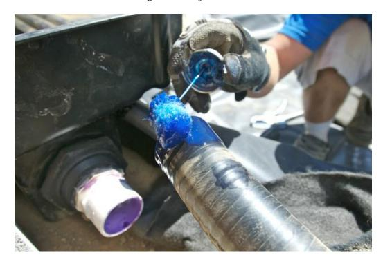
When the adapter fitting is securely fastened use the PVC primer and then the PVC glue on both the inside of the adapter and the outside of your tubing. Quickly insert the tubing into the fitting
