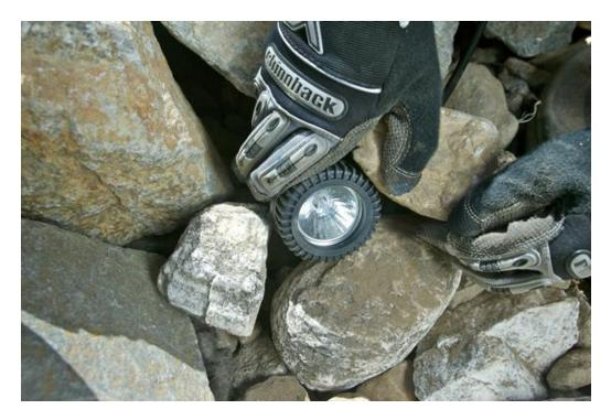
Try to place the light body in between two or more rocks pointing out. This will conceal the light from view during daylight hours. Lights at the base of the waterfall pointing up are popular and allow you to continue viewing the falling water after dark.
