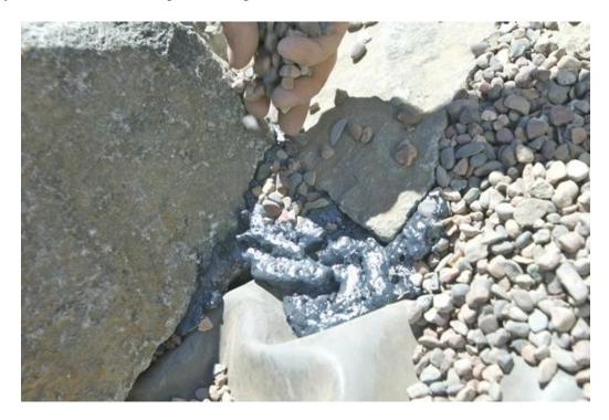
Use the can of rock foam that is included with your kit to fill in cracks between stacks of rocks. Use foam where flat rocks meet the liner to keep the water flowing above them.
