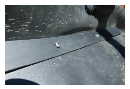
Once all bolts are in place, use a wrench to tighten each nut until the compression strip is snugly against the spillway. This procedure is done to ensure that the liner is sealed to the spillway. This will prevent water from leaking underneath the liner when the waterfall is running. Do not over tighten the bolts as cracking of the compression strip may occur. Tighten only until strip is snugly against the spillway.
